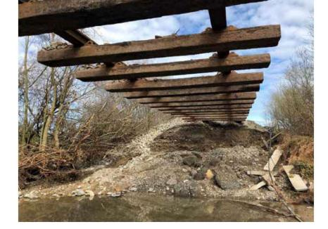
Work was also undertaken to ensure the track was safe, replacing and replenishing contaminated ballast, and after test trains ran through on Sunday evening to check the repairs and test the signalling, the railway was ready to open on Monday 18 February, one week after the landslip had occurred.
