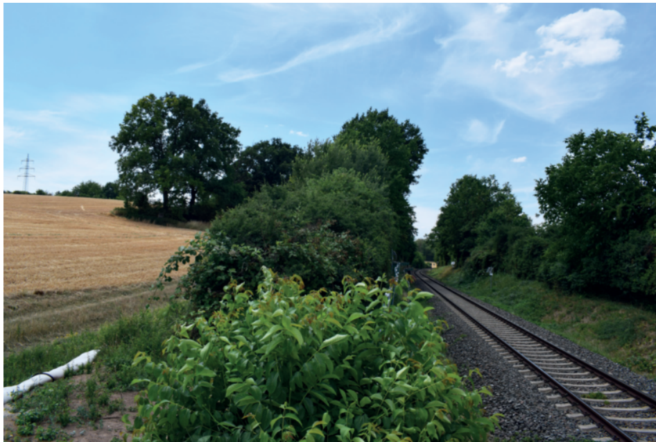
Test project near Eisenberg. The embankment (under the trees) is characterized by sandy soil, which is why sudden landslides are likely during heavy rain. Therefore, no laser sensors are installed.
