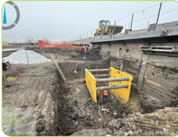
SoE system being installed adjacent to railway
